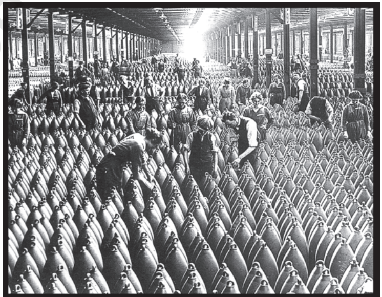
Fig. 20 – Workers in a munition factory during the First World War. Production of armaments increased rapidly to meet war demands.
